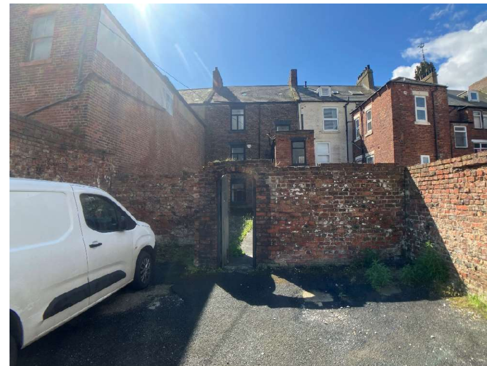
Figure 4.1. – External image from service road to northwest of site.
