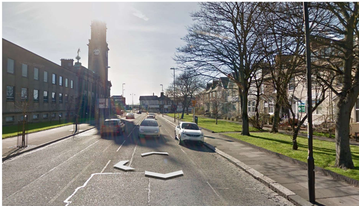
Figure 3.1.02 – SouthEast view, showing impact of the Town Hall against the terraced housing.
